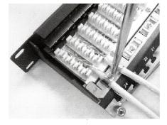
Fasten the screws through metal case to hold tightly down for two cable jackets in the same time.
