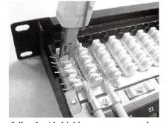
Press foil or braid shield to contact ground, and keep the cable straight;
