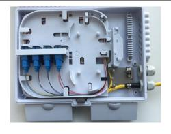
Pass the spliced pigtails to the upper side of the tray and
